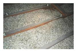
Largely, the non-asbestos vermiculite attic insulation comes from South Africa. This is somewhat larger in size than Zonolite. There were also attic insulation products sold that included a mix of Zonolite and South African Vermiculite.
